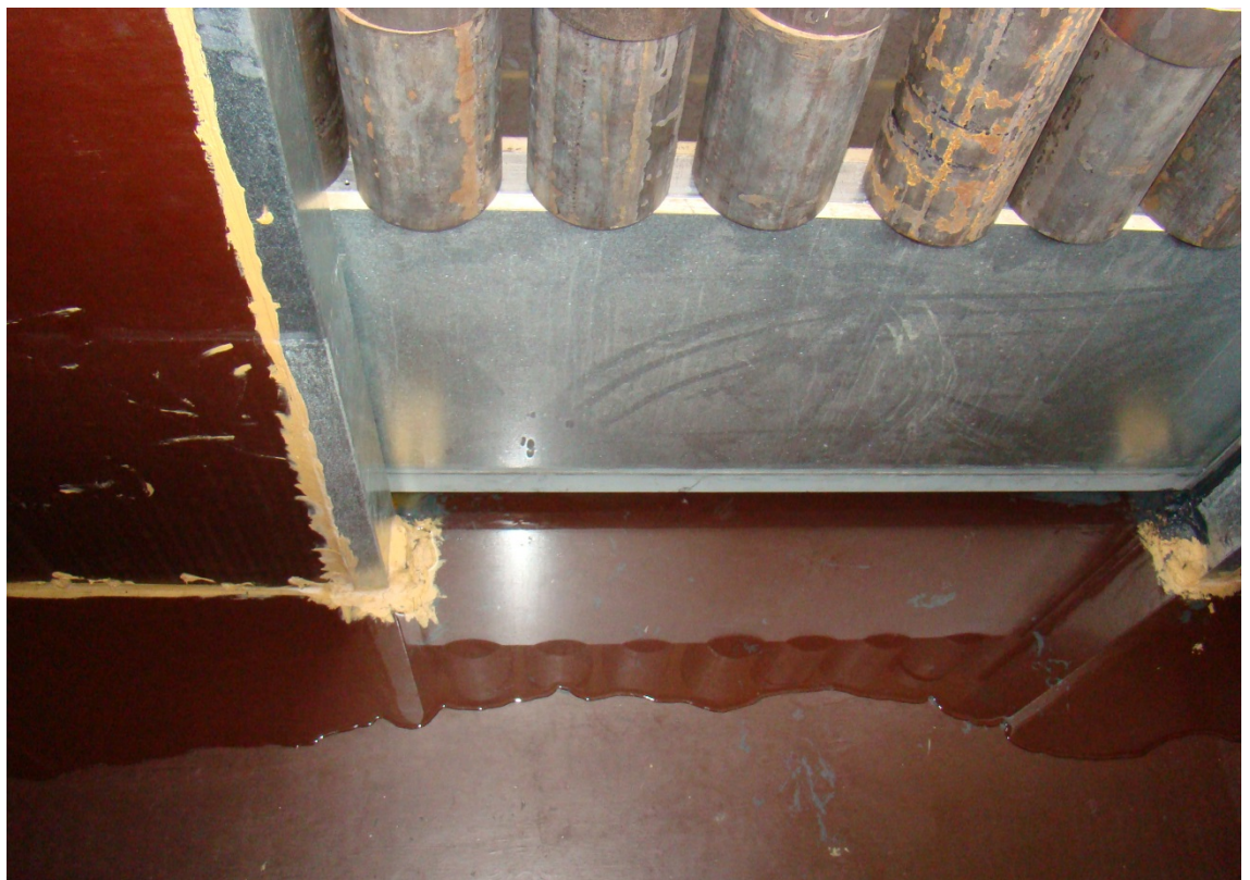
Photo C.6 Leakage under the specimen 500 mm, water at outside
